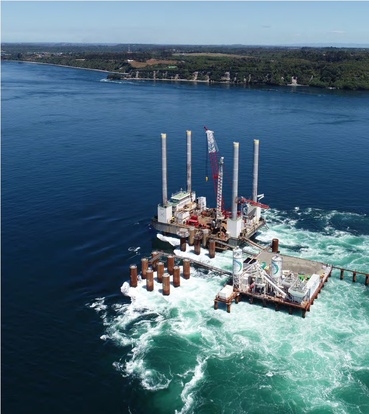
Foundations works for the Chacao Bridge, Chile
