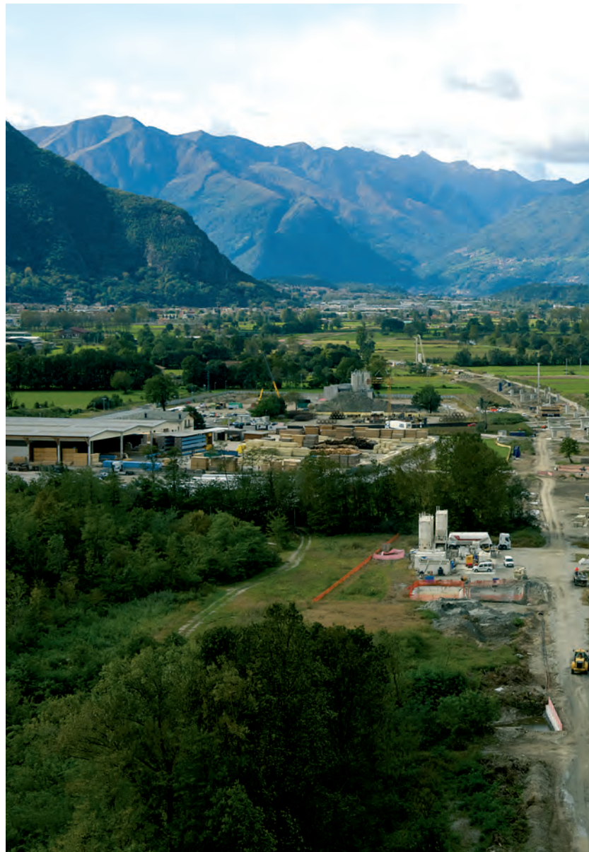
Foundation works for the Pedemontana - Italy motorway
