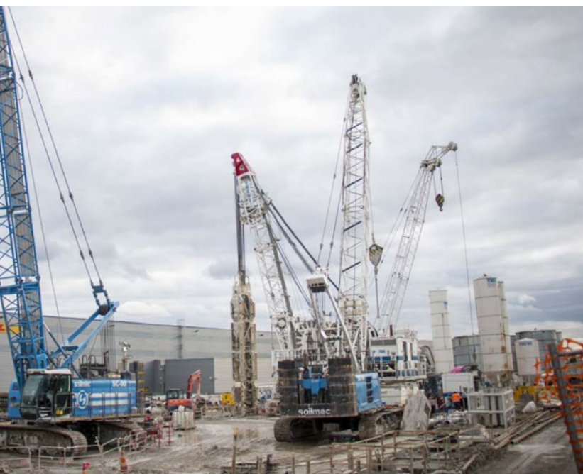
Foundation works for the "Grand Paris Express" Project _ France
