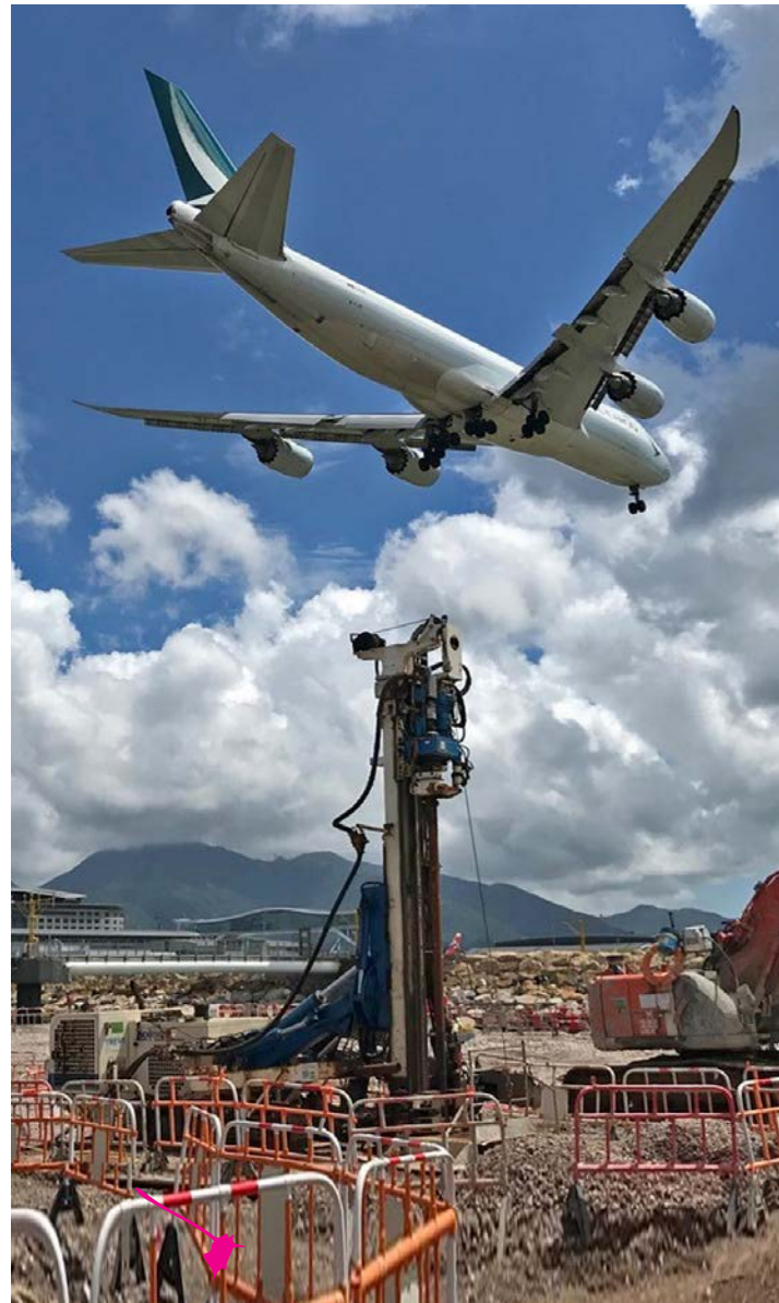
Consolidation works for the new Hong Kong airport
