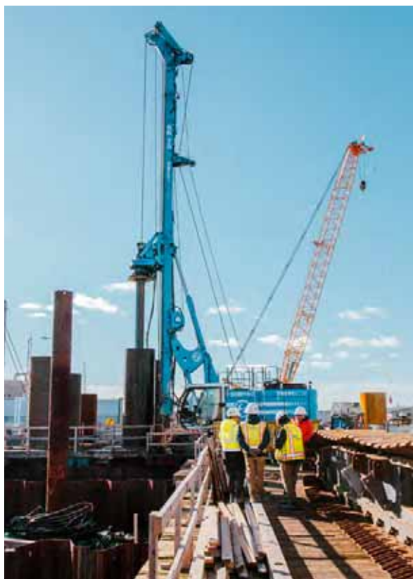
Belden Bly bridge project / MA, USA
