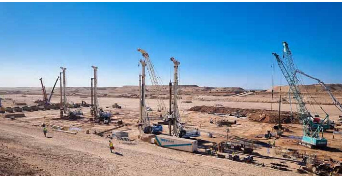
NEOM, the Line project | Cantiere Trevi | Arabia Saudita
