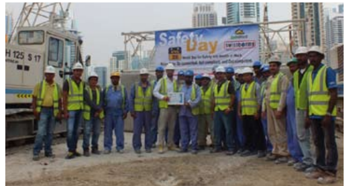
Swissboring Capitol Tower project
