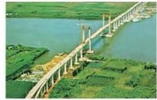
**Bridges on the Paraná River in Argentina**, for the first time a company executes piles in the water to a depth of 74 meters
