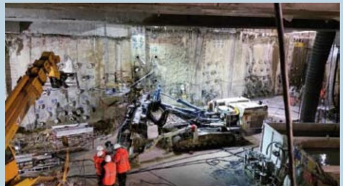
Metro C of Rome – San Giovanni station – under-crossing of existing station line "A". Soil consolidation works executed with injections and ground freezing.
