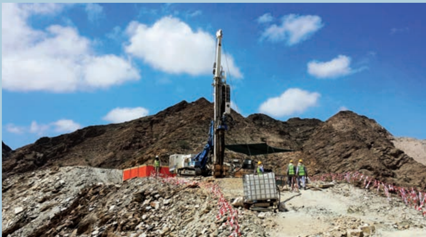
Indagini geologiche per il “Sifah Road Project”./Soil investigation for the “Sifah Road Project”.
