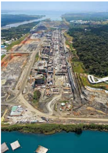
Vista aerea del cantiere. Aerial view of the yard.
