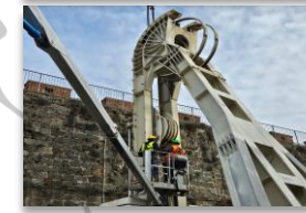
Securing the Garisenda Tower in Bologna
