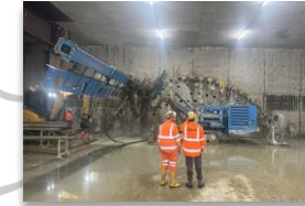
Florence High-Speed Rail Link (PNRR)
