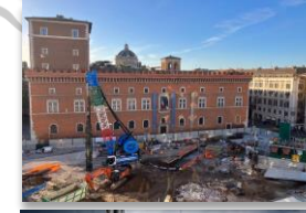
New Piazza Venezia metro station - Line C
