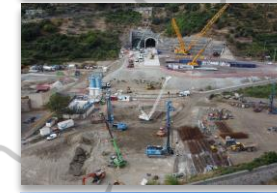
Messina - Catania railway doubling
