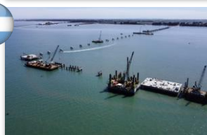
Dock Oiltanking Puerto Rosales
