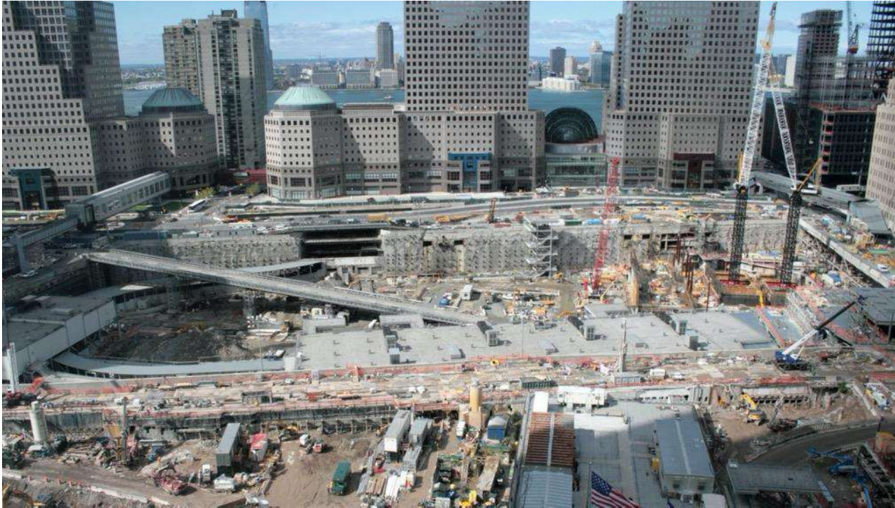
Foundation works for the reconstruction of the World Trade Center and metro station
