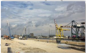
Terminal container Montesyndail - Venezia
