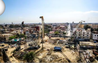
Baraki metro and railway station (Algeria)
