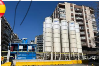
Extension of metro line 8 in Barcelona (Spain)
