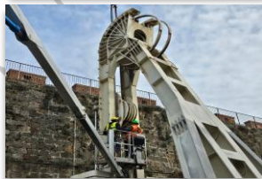
Securing the Garisenda Tower - Bologna
