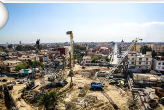
Baraki metro and railway station (Algeria)
