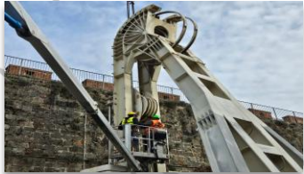
Securing the Garisenda Tower - Bologna
