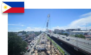
South Commuter Railway Manila (Philippines)
