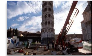
Consolidation of the Leaning Tower of Pisa (Italy)
