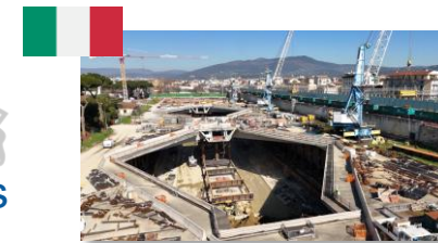
High-Speed Rail Link (PNRR) (Florence)
