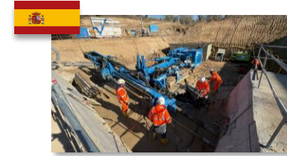
Extension of metro line 5 in Madrid (Spain)
