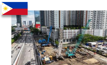
Metro Manila Subway (Philippines)
