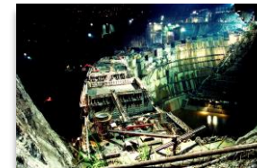
Ertan Dam (China)
