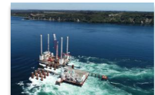
Chacao Bridge (Chile)
