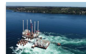
Chacao Bridge (Chile)
