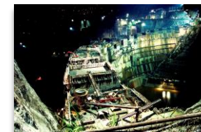
Ertan Dam (China)
