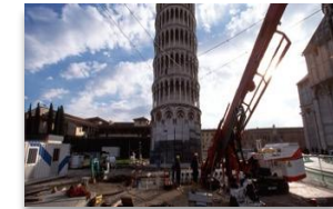
Consolidation of the Leaning Tower of Pisa (Italy)
