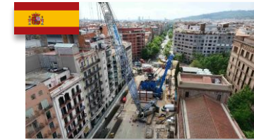
Extension of metro line 8 in Barcelona (Spain)
