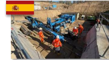
Extension of metro line 5 in Madrid (Spain)
