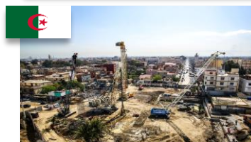
Baraki metro and railway station (Algeria)
